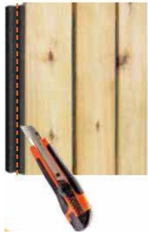
Fig 7. Using a utility knife or skill saw, remove the rubber side support by first scoring it, then go over the same cut again to completely separate the rubber side support from the base.
